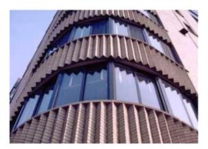
The historic steel sash (see photo above) was removed and replaced with modern aluminum sash, resulting in a negative visual impact on the building's historic character. Photo: NPS files.
