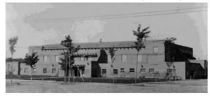
building was substantially rehabilitated in 1982, including re-roofing and stucco repair, and although the interior space was subdivided, it still retains its original brick walls, maple gym floor, and vaulted metal trussed roof.
